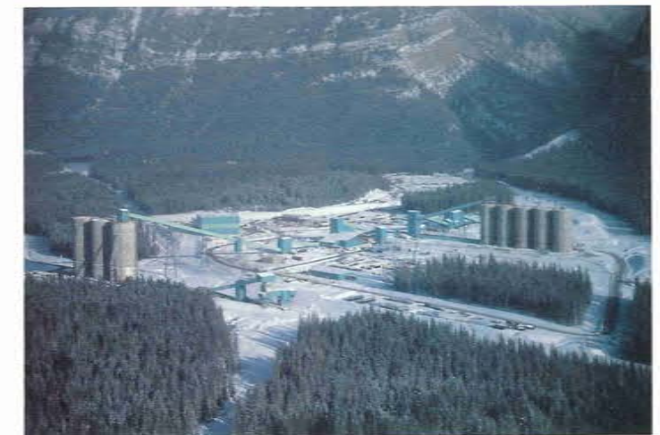
▼ An aerial view shows the processing plant with the load-out silos on the left and raw coal storage silos on the right.
